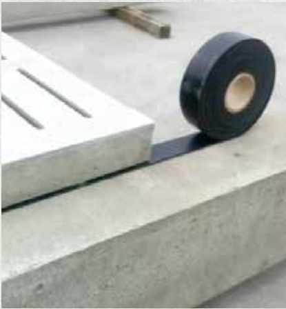
Rubber base for height adjustment
